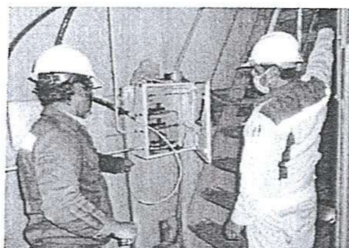
Flushing Sampling tube for Heated line stack1,2
